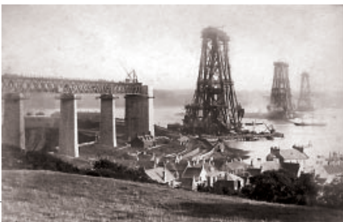
The bridge during construction showing the height of the cantilever towers
