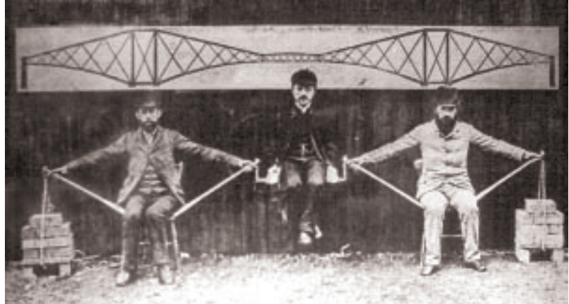
The cantilever principle had to be demonstrated to give the public confidence in the design
